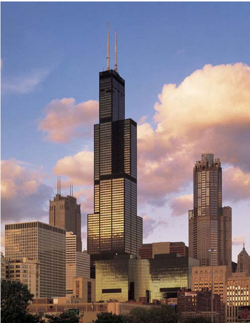
Chicago – [redacted] tallest building in the USA
